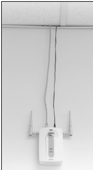
Figure 9 Run the Cables Upward
